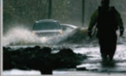
Water main break on River Road
